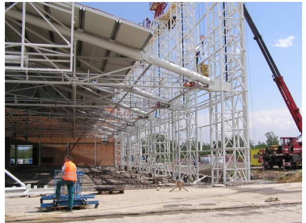
Fig. 12: Lifting of the roof
