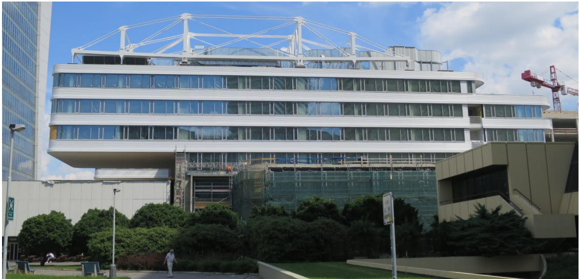
Fig. 17: Suspended concrete structure of Trimaran
