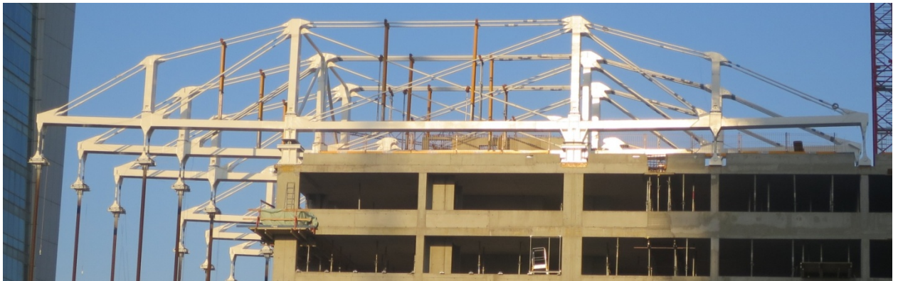
Fig. 18: The trio of three truss girders
